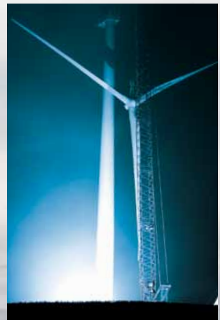
The last turbine was topped out the night of Dec. 4, 2009.
