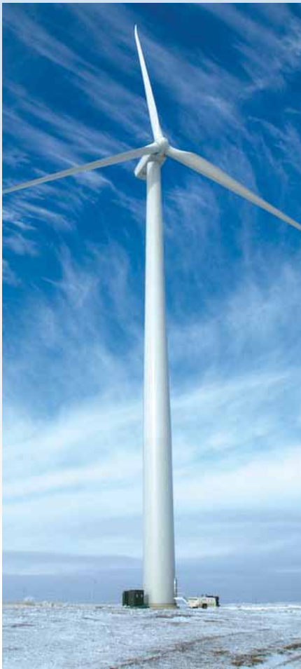
PrairieWinds 1 is the nation's largest wind project owned solely by a cooperative. Its 77 turbines dot the landscape between Minot and Max, ND.
